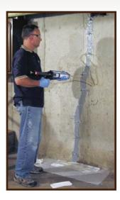
Cracks in the foundation are all too common. While they seem to pose no immediate threat, the fact is, most foundation cracks have the potential to grow wider and cause serious problems down the line. Most foundation cracks form as a result of shrinkage from excess water within 28 days after the concrete was initially poured. Through time, foundation cracks typically grow larger, resulting in a greater opportunity for water seepage or the possibility of structural deficiencies.
